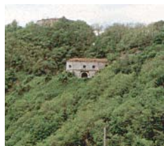
The tunnel under the Forte di Altare. On the facing page, the milestone that marks the beginning of the Alps and, at the bottom, the Forte Baraccone.
